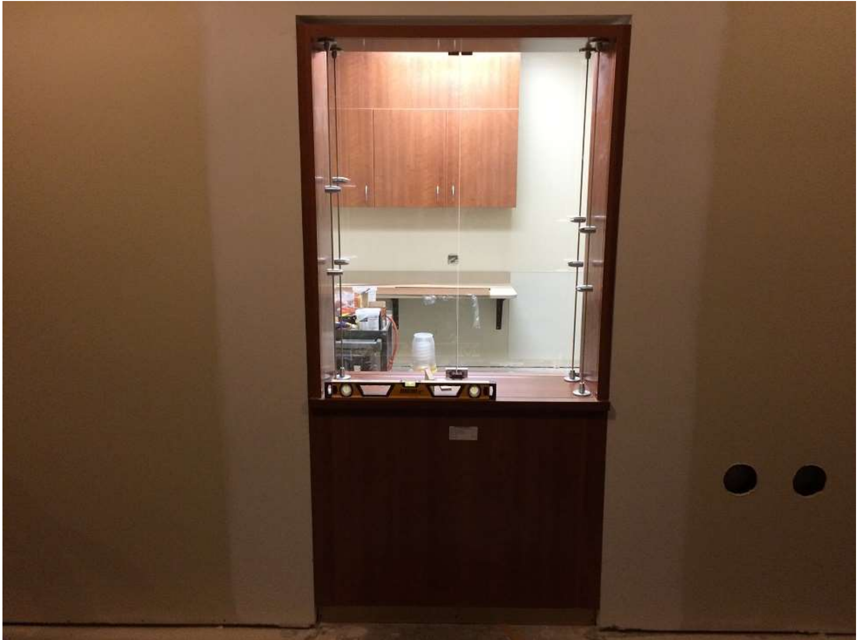
Millwork installed first level.
