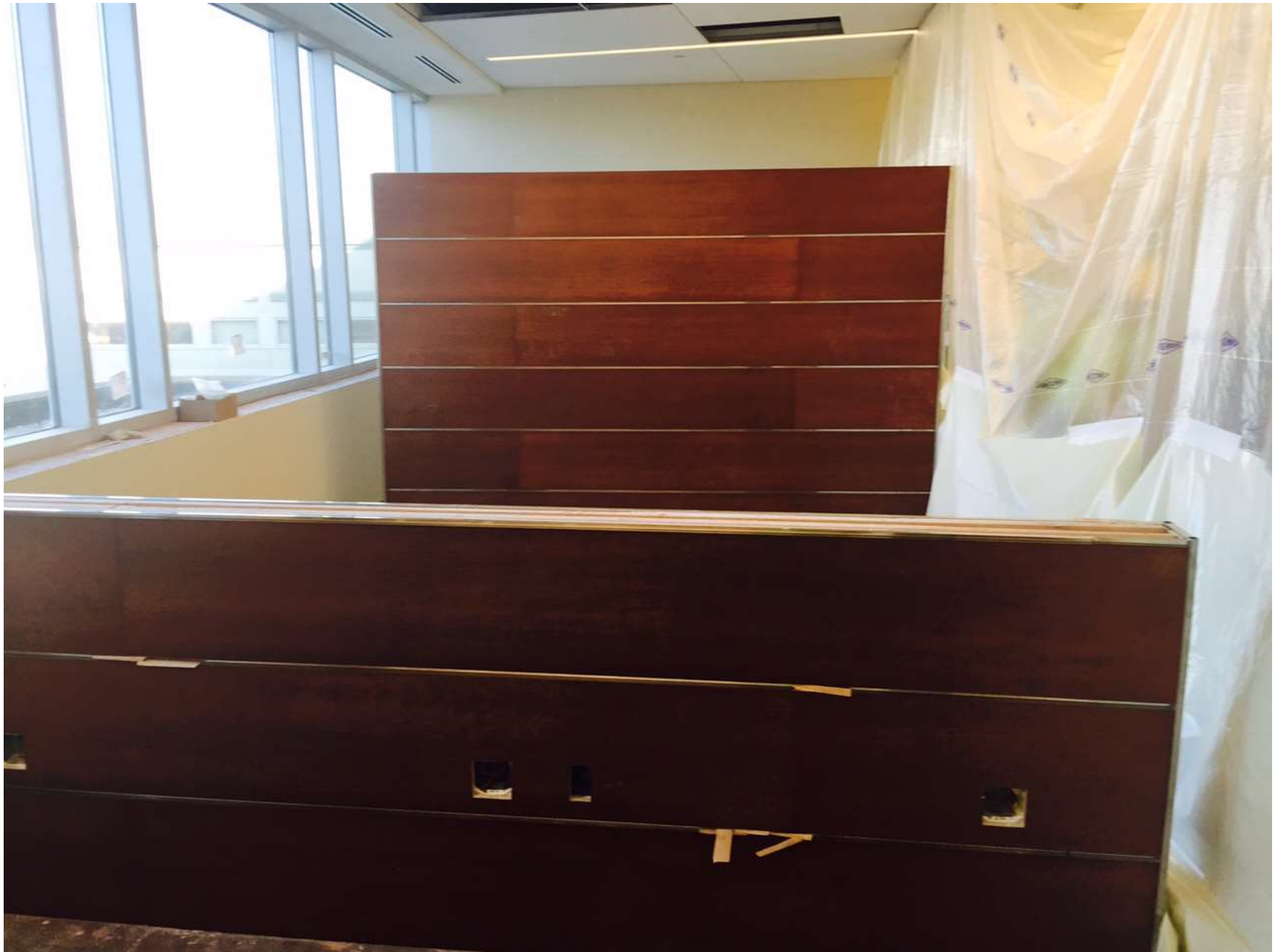
Interior Wood Paneling on Second floor.
