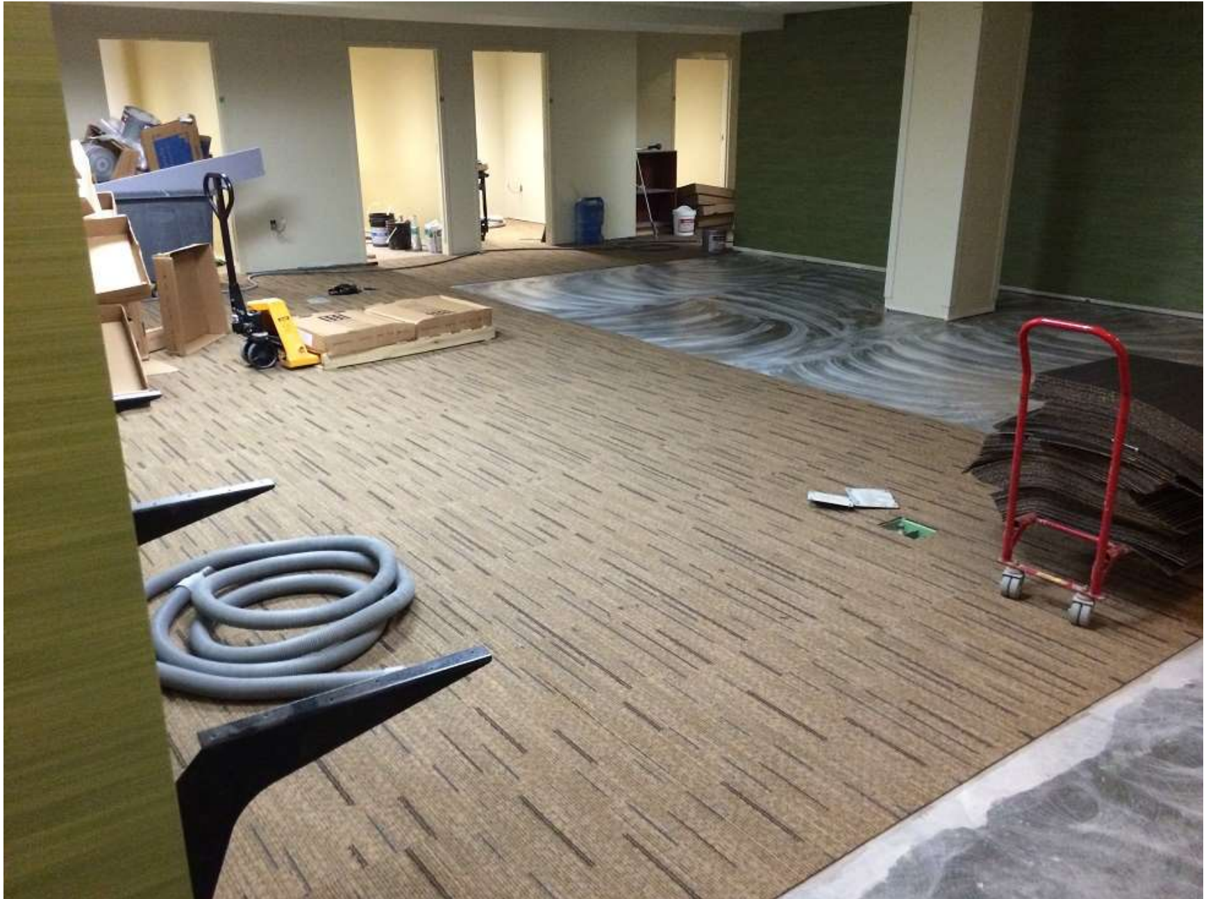
Carpeting being installed first level.
