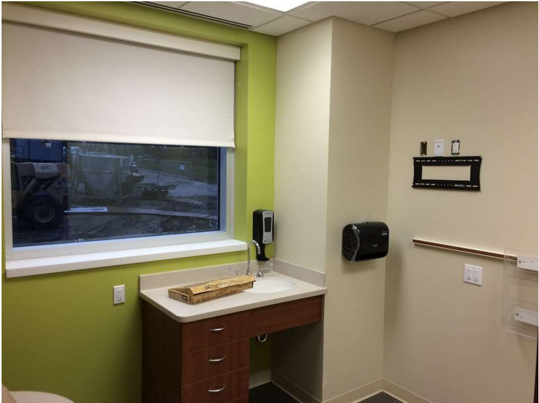
Wall mounted items and blinds installed second level.
