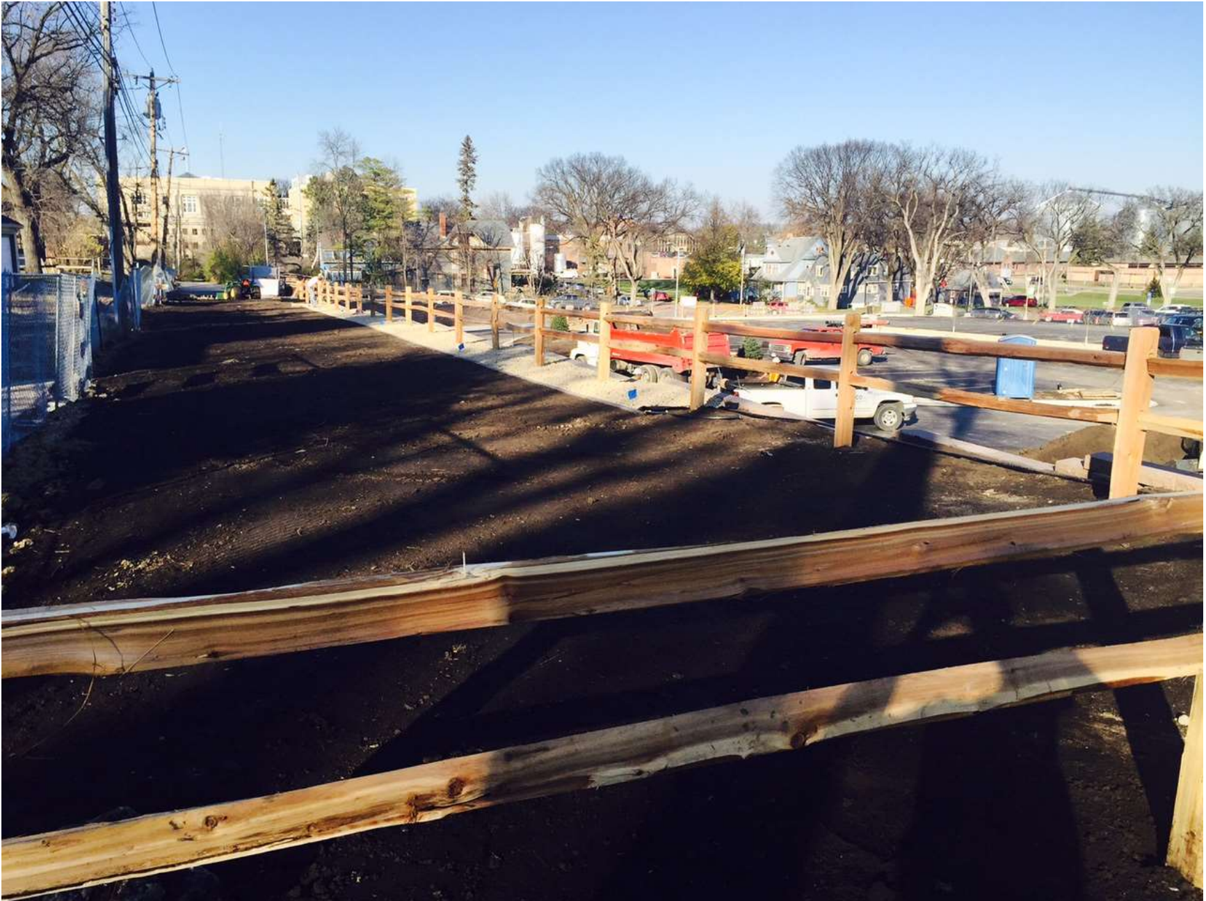
Fencing and Landscaping along North West Retaining wall.
