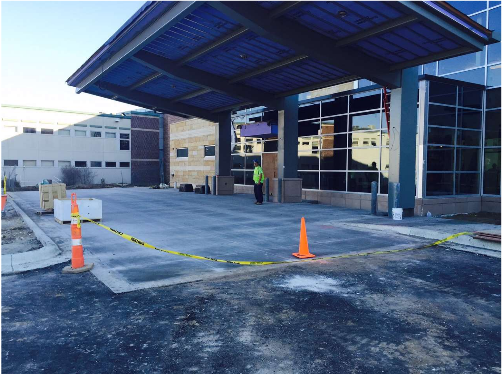
Entry Snowmelt apron poured.
