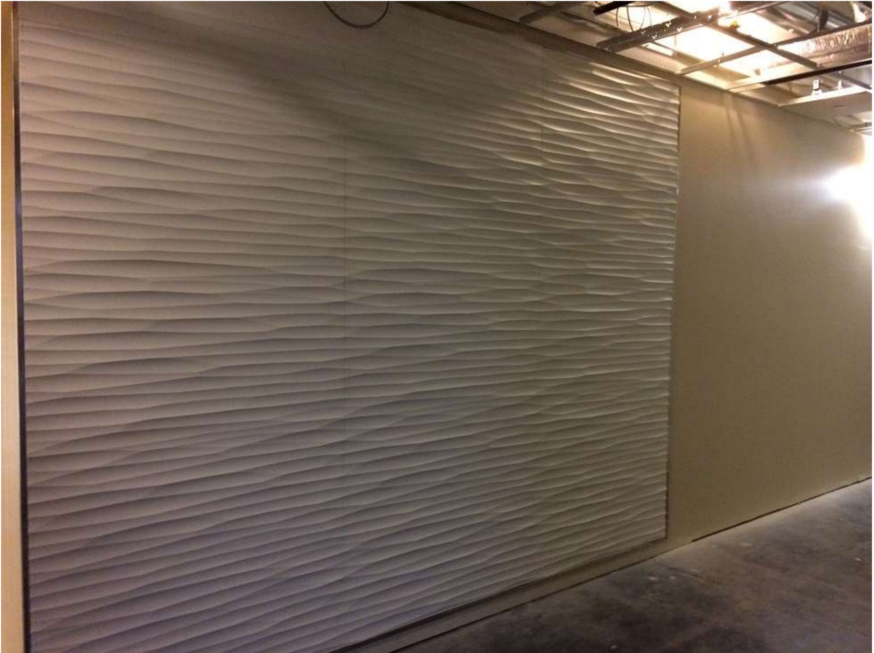
Decorative wall Paneling installed.
