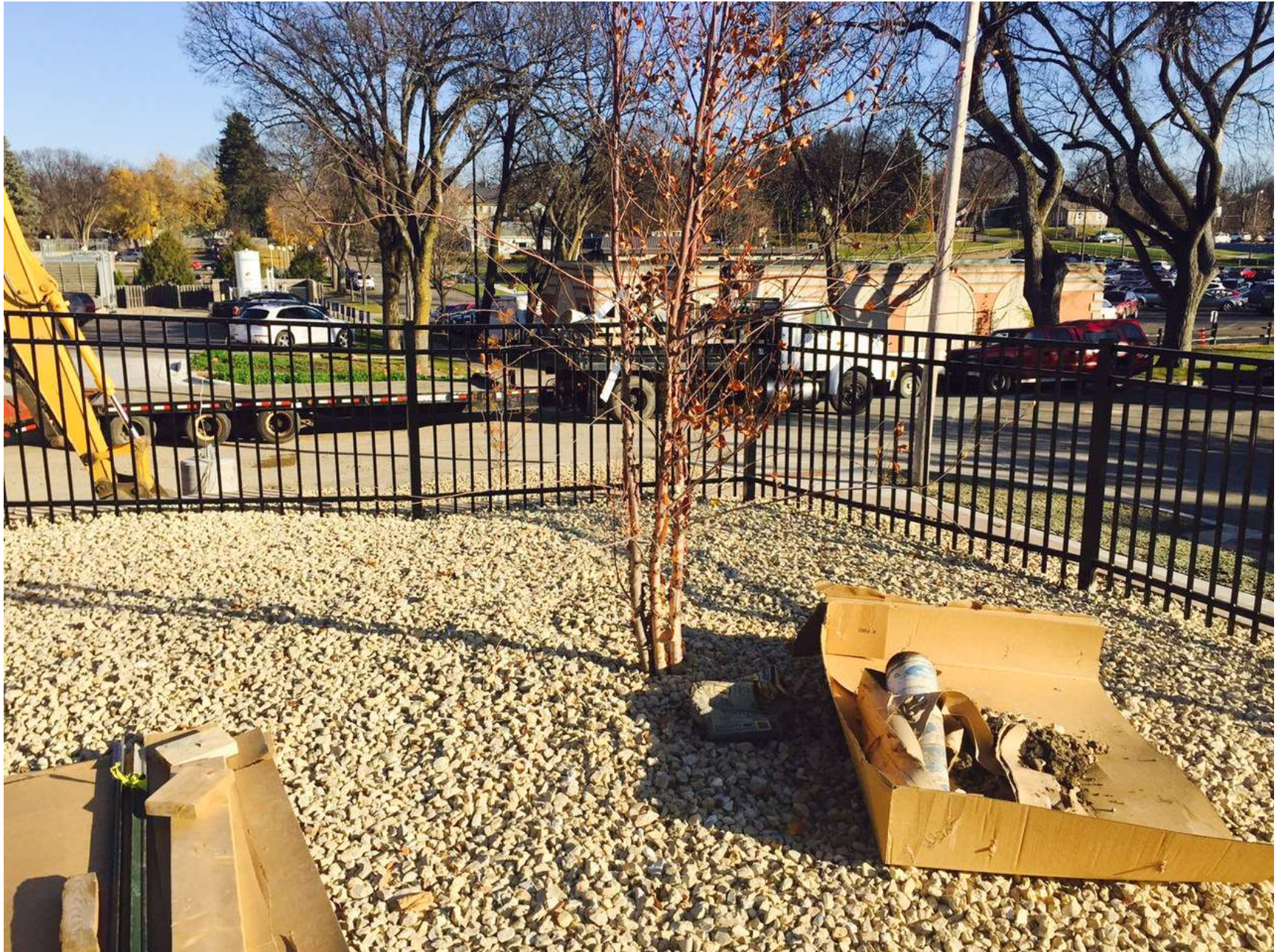
Landscaping and Railing on South side of Clinic.
